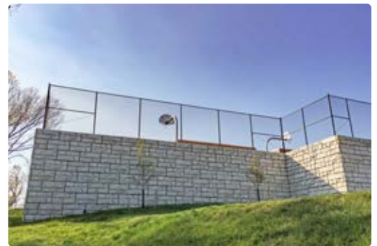
Takoma Park Middle School - Takoma Park, MD
