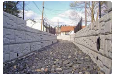
Municipal Drainage Projects
